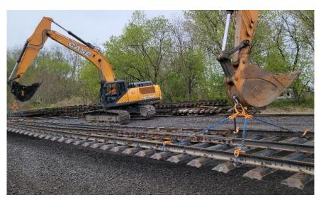
"The steel tie is resistant to damage, corrosion and deterioration. It's 100% recyclable making it the superior option for usage in a busy rail yard such as Geneva," states Joann Armstrong-Bruch, General Manager of Finger Lakes Railway.
